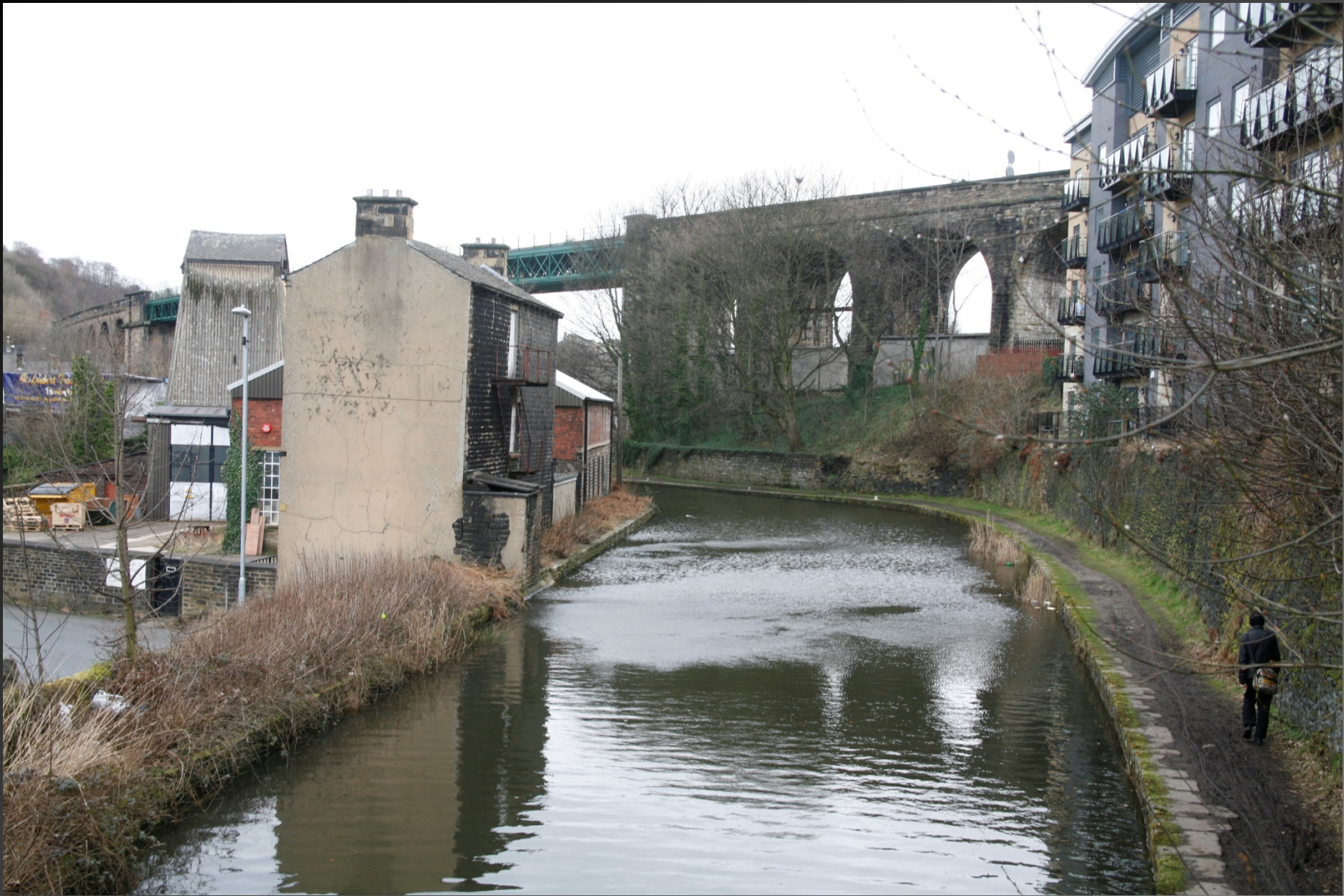
Site Of Fisher's Cropping Shop
