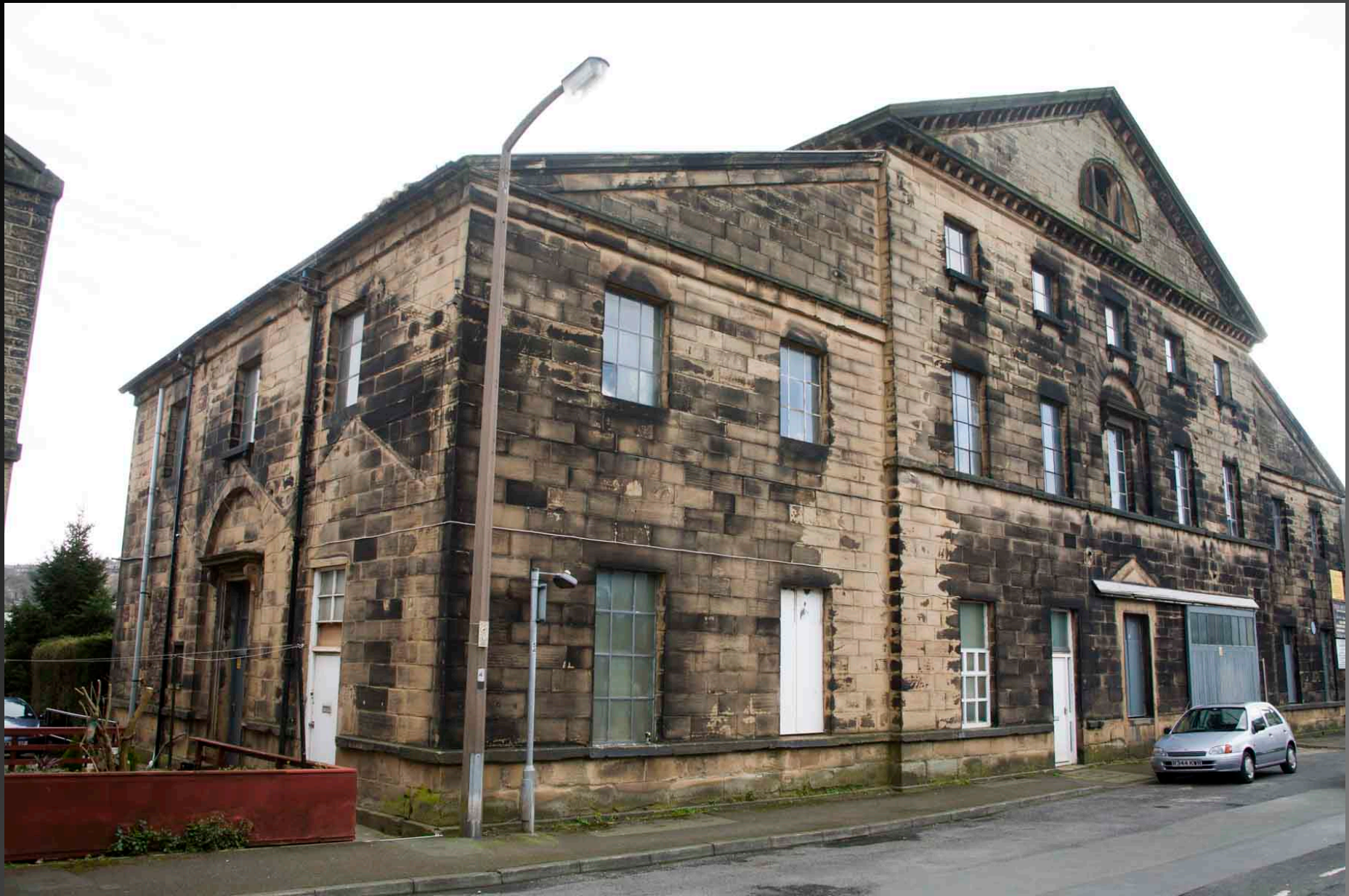
Milnsbridge House - front
